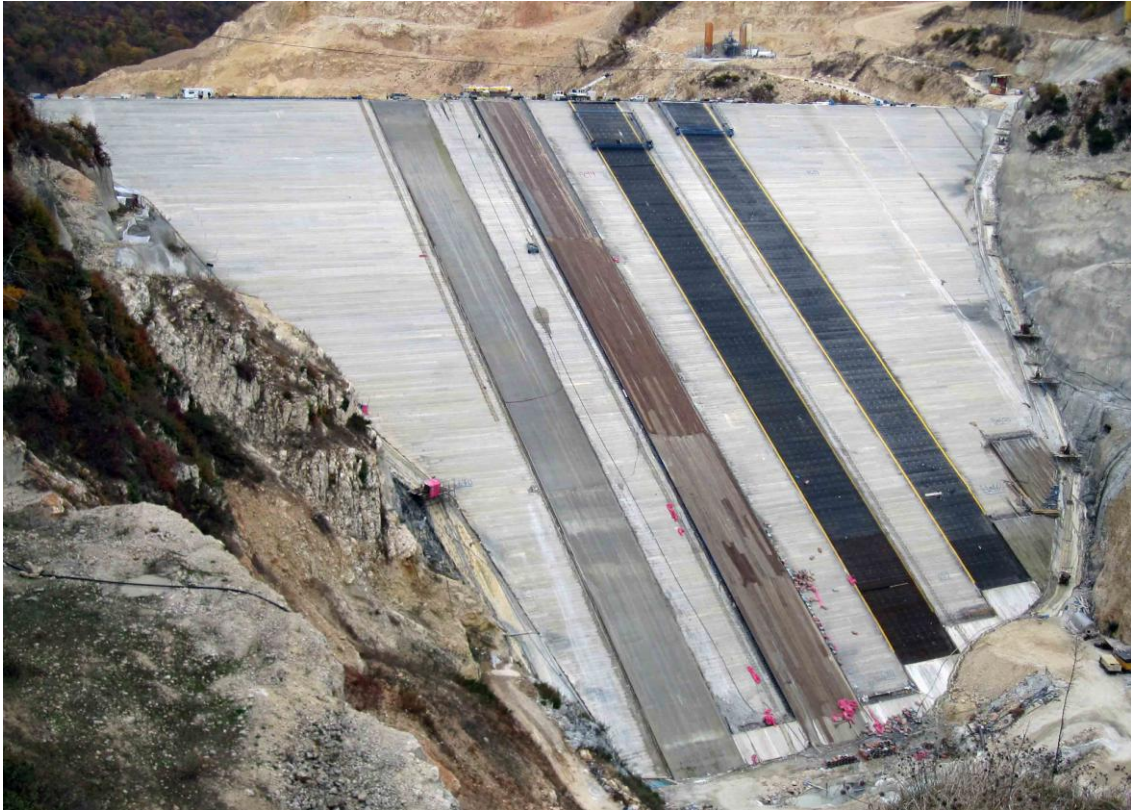
Figure 5: Concrete face of Gelevard dam
